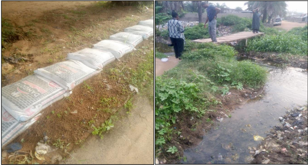
Figure 3. (i) Sandbags used in flood mitigation; (ii) Wooden Bridge made by locals.
